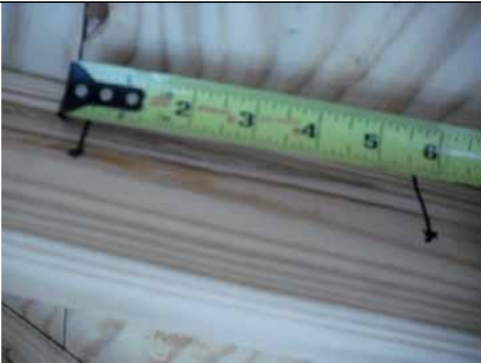
Roof deck attachment
