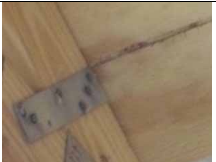
Roof to wall attachment
