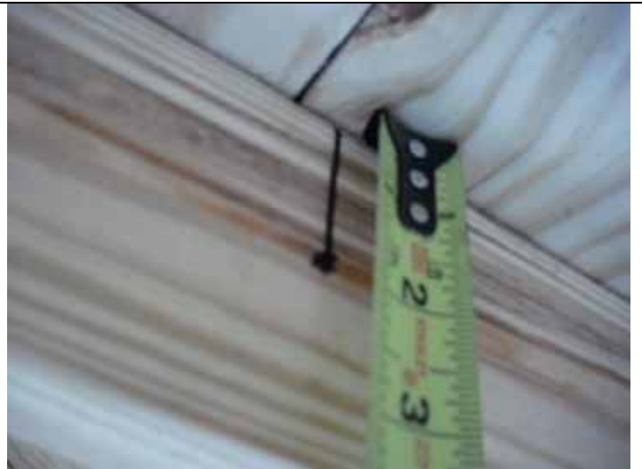
Roof deck attachment
